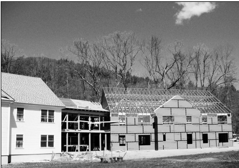
The new Bob & Virginia Barrett Wing takes shape
